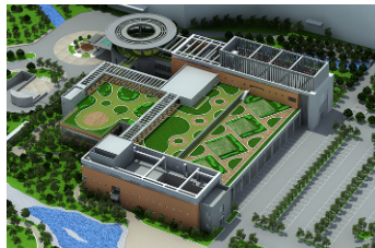
Chang Gung Memorial Hospital, Kaohsiung (Kaohsiung, 2018)
