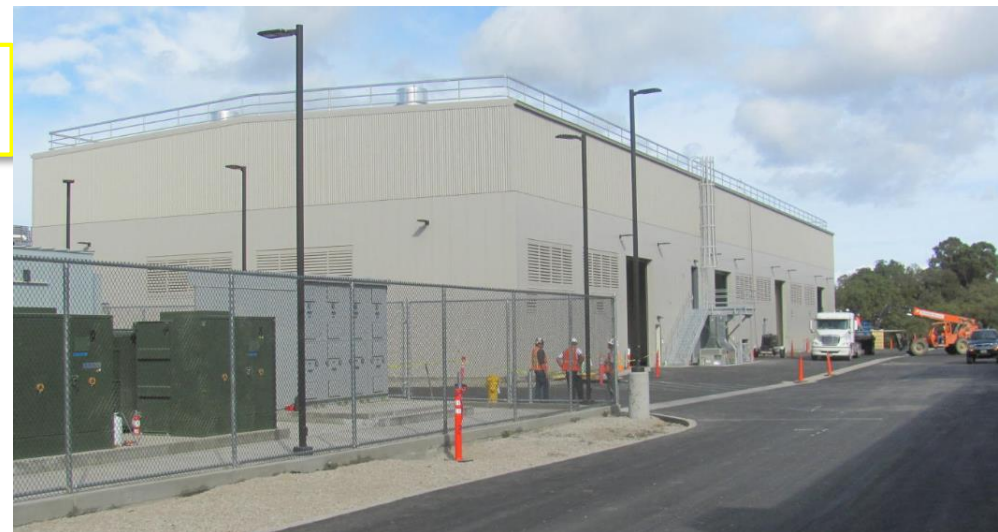
CryoPlant Building at Sector 4
