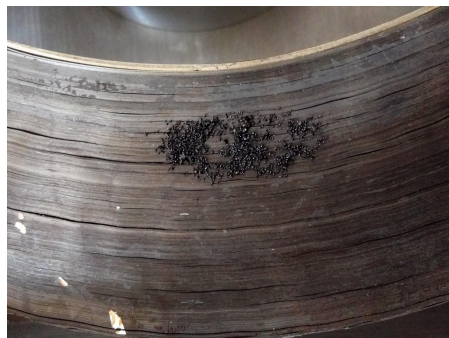
Figure 8: Local damage of type A MA core.
