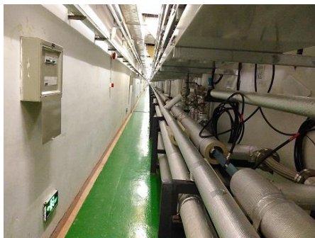
Figure 3: The 324MHz reference line of the CSNS Linac.
