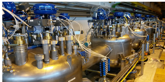
Figure 1: Cryogenic distribution line feeding the SC linac with liquid He at 4.5K.
