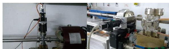
Figure 5: FS installed in TL 2 (left) and motorized one in SR injection section (right).
