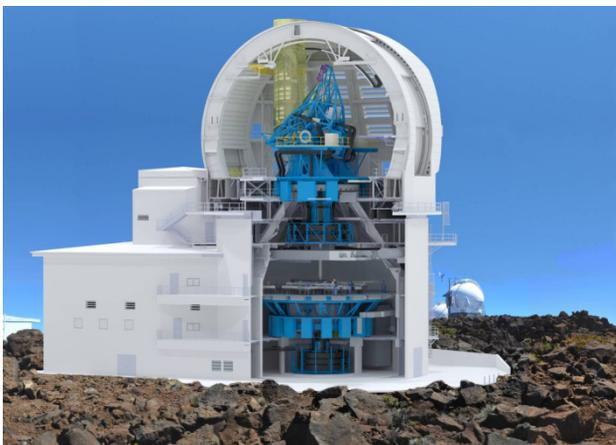
Figure 1: Cut-away image of telescope enclosure showing the telescope and coude rotator.
