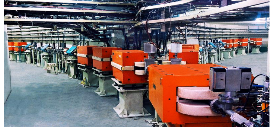
crossing of the transport line
