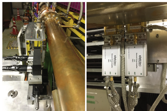
Figure 1: The top of the pillar holding the sCVDs and the ZDLM monitors downstream from the IP in the LER on l.h.s and the sCVDs connected to the charge amplifiers in the HER on r.h.s.
