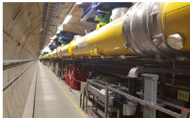
Figure 1: XFEL tunnel view.
