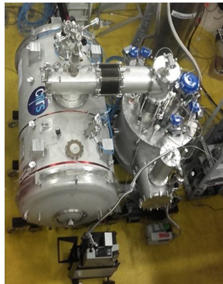
Figure 1: Picture of ESS prototype spoke cryomodule with its valve box, installed in the test pit at IPN-Orsay.
