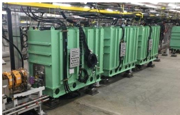
Figure 6: \beta = 0.041 CMs after installation and alignment in the FRIB tunnel.
