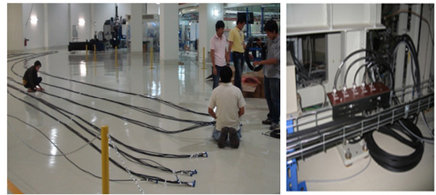
Figure 3: Installation of the new BPM signal cables.
