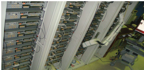
Figure 3: Set up for the acceptance test.
