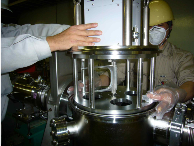
Figure 2: Installation of the horizontal flying wire monitor.
