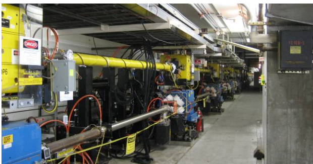
Figure 3: LER vacuum chamber in IR12 (upper beam pipe). The outer clearing solenoid can be seen.
