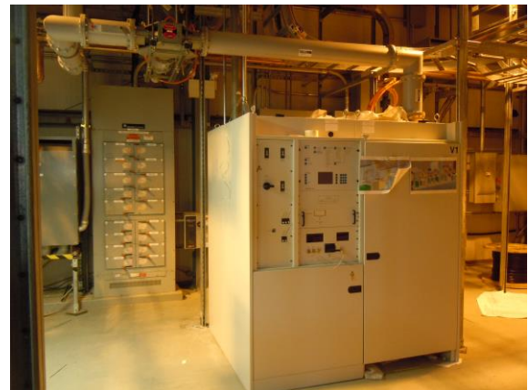
Figure 9: 500 MHz power amplifier for CeC PoP.
