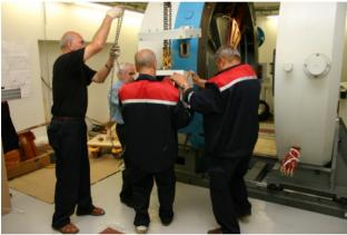
Figure 2: The NIIEFA team installing the matching dipole. The cyclotron magnet opens sideways on precision rails.
