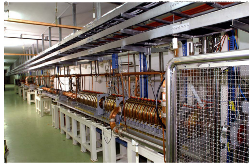
Figure 1: The tunnel of SDUV-FEL
