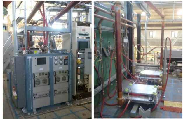
Figure 6: The 186 MHz CW 120 kW RF system. The tetrode-based amplifier (left), and the two circulators situated in the two branch lines (right) are visible.
