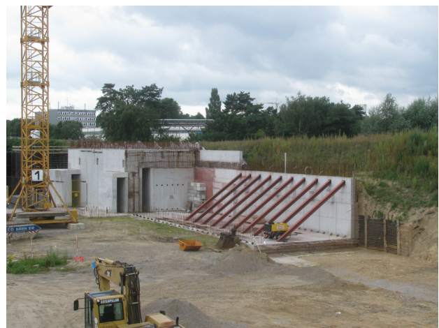
Figure 3: FLASH2 construction site August 2012.
