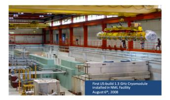
Figure 12: Installation of a US-assembled 8 cavity TESLA cryomodule in the New Muon Laboratory facility at Fermilab.
