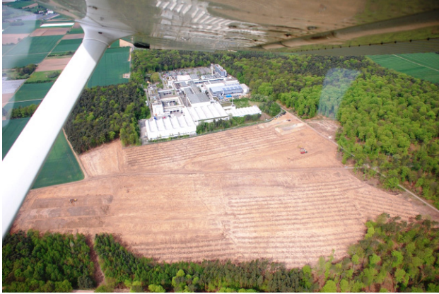
Figure 4: Clearing of the first section of the FAIR construction site.
