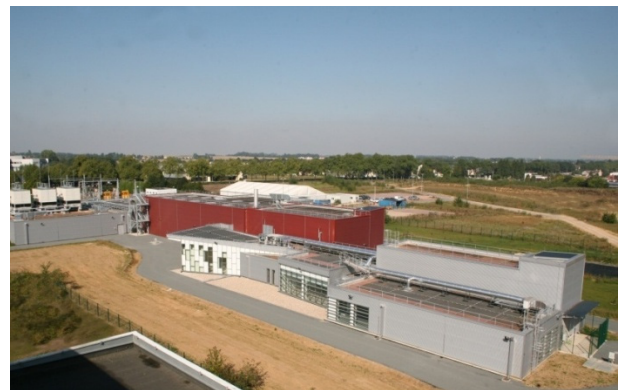
Figure 2: Completion of the accelerator building (October 2014). The beam axis is 9.5 meters underground.
