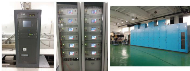
Figure 8: Superconducting spoke cavity power source (left), superconducting magnet power source (middle), RFQ cavity power source (right).
