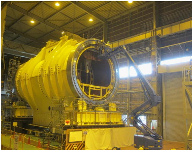
Figure 5: Rotation tests of the gantry structure at the Toshiba Keihin Product Operations.
