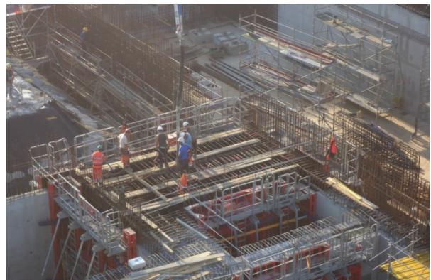
Figure 9: Iron mesh of the SPIRAL 2 building.
