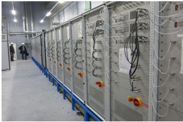
Figure 6: Solid state 88.0525 MHz amplifiers.
