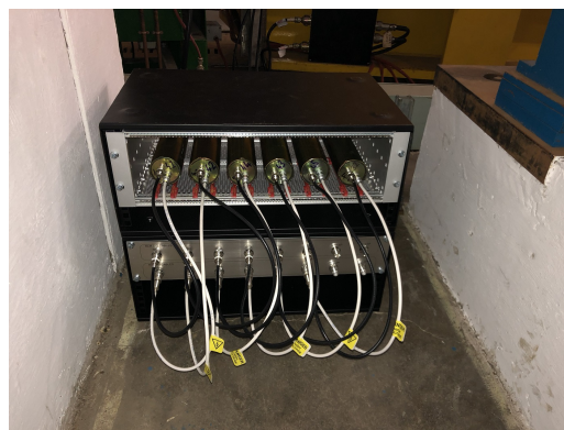
Figure 5: Chassis to house PMTs for a single dipole.
