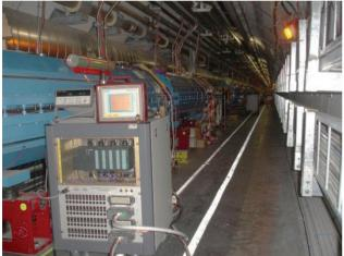
Figure 2: Bake-out mobile cabinet in the LHC Tunnel.
