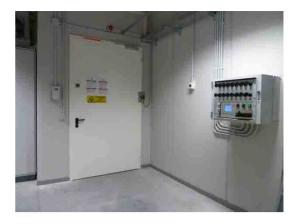
Figure 3: The badge reader and baton panel next to the linac door.
