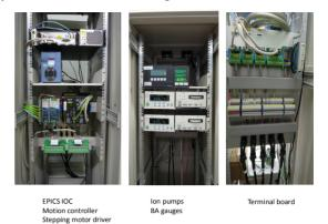
Figure 4: Control rack layout of IU22 for TPS.
