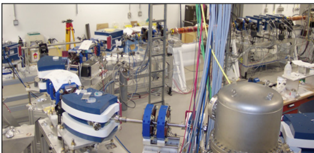
Figure 5: Installation of the isochronous bend leading to the MIR wiggler. The accelerator is in the upper background right and the diagnostic beamline exits at the top left.
