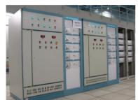
Figure 5: Storage ring Q power supplies for one station
