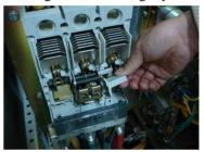
Figure 8: The contactor handle was broken
