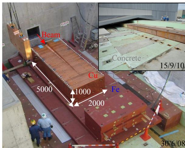
Figure 1: The beam dump at Hadron hall (under construction).
