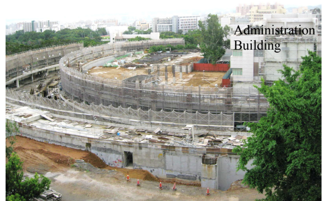
Figure 2: Status of the TPS ring construction.
