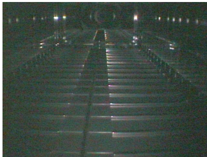
Figure 3: Photograph of inside of the kicker magnet.
