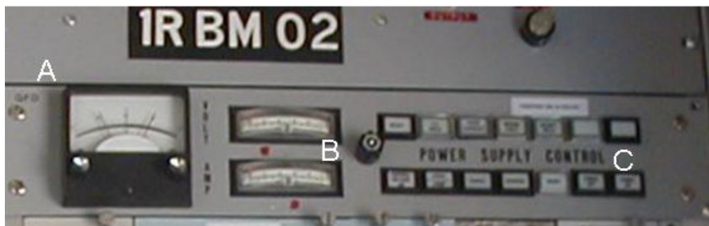
Figure 2: LAMPF-Standard power-supply controller circa 1970. (A) – Ground-Fault Meter with trip setting. (B) – Output Current and Voltage (C) – Integrated control switches and indicators. Picture taken 2003
