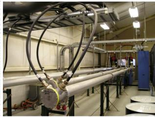
Figure 1: RHIC injection kicker Blumlein triaxial pulse generators.
