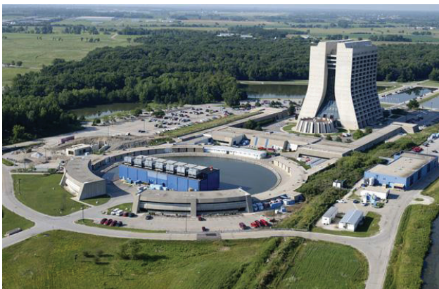
Figure 1: Fermilab’s Booster synchrotron
