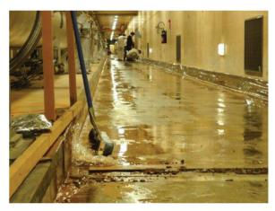
Figure 2: Inflow water into the tunnel.
