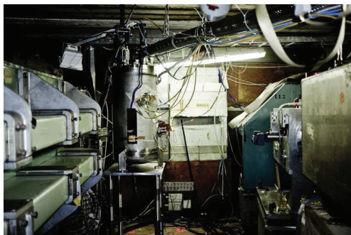
Figure 2: Cryostat and liquid helium transfer line installed in the active zone.
