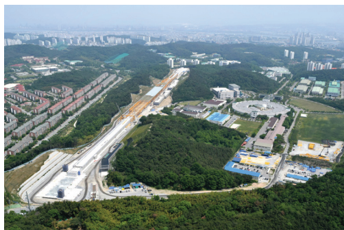
Figure 1: Construction site of PAL-XFEL.
