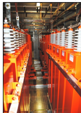
Figure 2: New power grid filter for SIS18.
