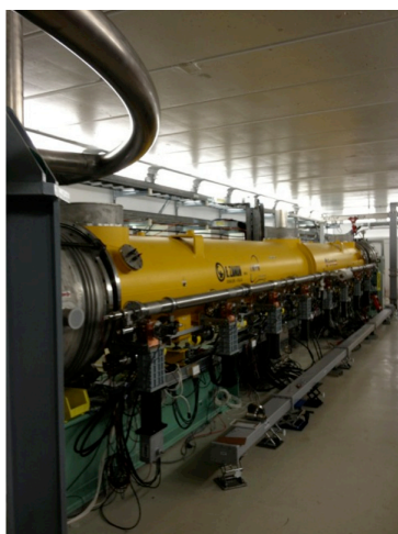
Figure 2: Cryomodule 2 installed in ASTA.
