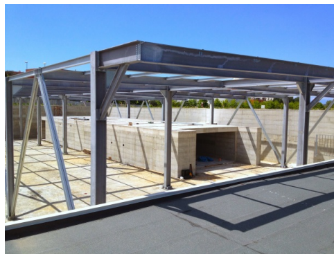
Figure 1: The project Hangar and the STAR bunker.
