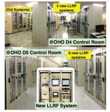
Figure 3: Installation appearance of the new LLRF control systems in the RF control rooms at D4 (upper) and D5 (lower) section.
