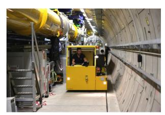
Figure 2: Cryomodule transport into the XFEL tunnel.
