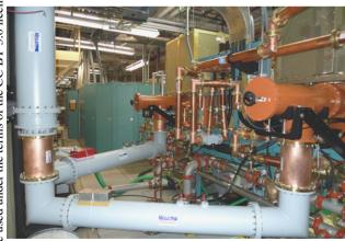
Figure 2: Coaxial feeders from PAs to branch hybrid.
