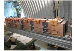
Figure 7: The kicker with Cu cooling plates in the RHIC tunnel.
