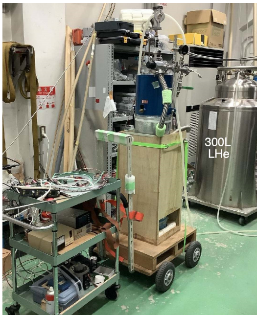
Figure 9: Experimental room at RCNP.
